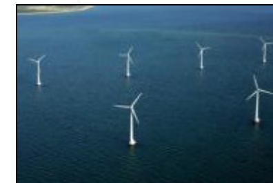
Electricity from wind power
